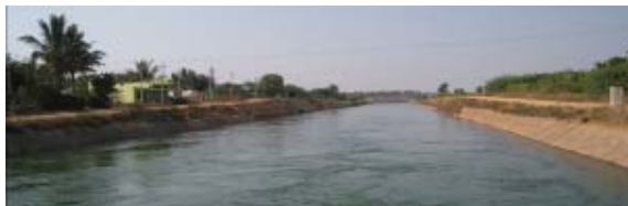
The Tungabhadra Left Bank Canal. Photo: David N. Barton
